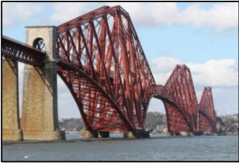
Forth Rail Bridge
